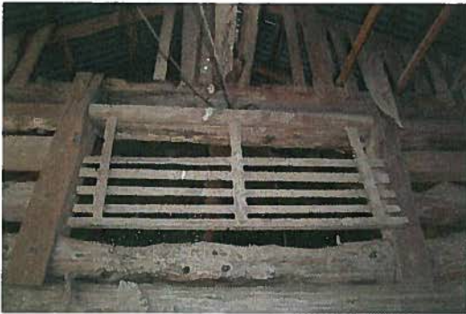
Crib door in upper wall of log barn, May 2008.
