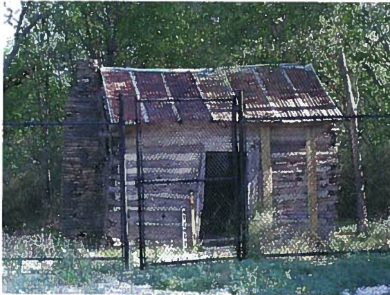
Log cabin with reinforcement, August 2007.
