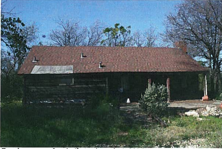
Farmhouse, east façade (facing log cabin), 200.9
