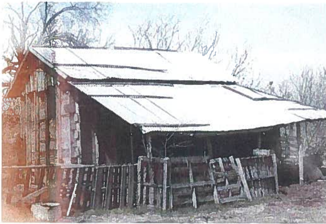
Plank barn, March 1973, shows barn's appearance prior to collapse. Photo by ARCHITECT WILLIAM THOMAS ODUM
