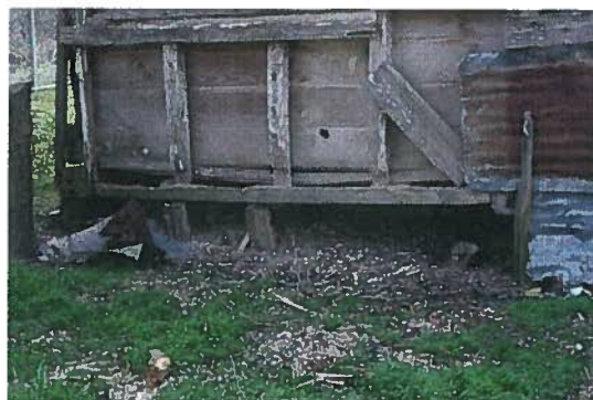
Log barn – details of crib with bois d'Arc piers, February 2008.
