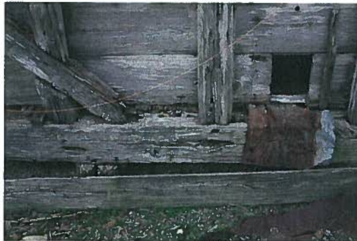
Log barn foundation at crib, February 2008.
