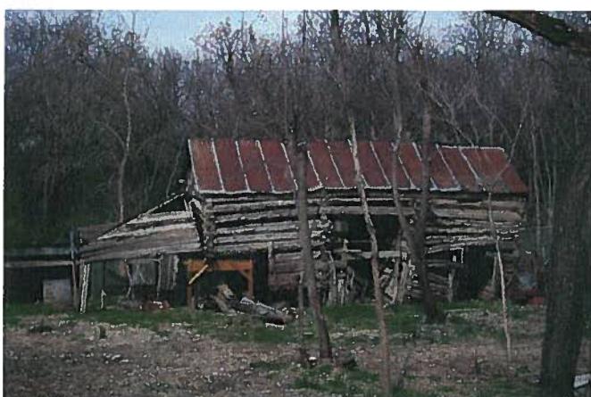
Overall view of the log barn with lean-to at left, February 2008.
