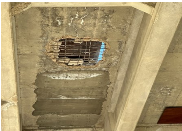
Example of emergency repairs done on SH356 Bridge
