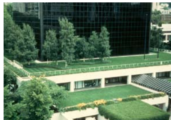
Rooftop gardens soften the urban environment and can provide usable open space for accommodating runoff.
