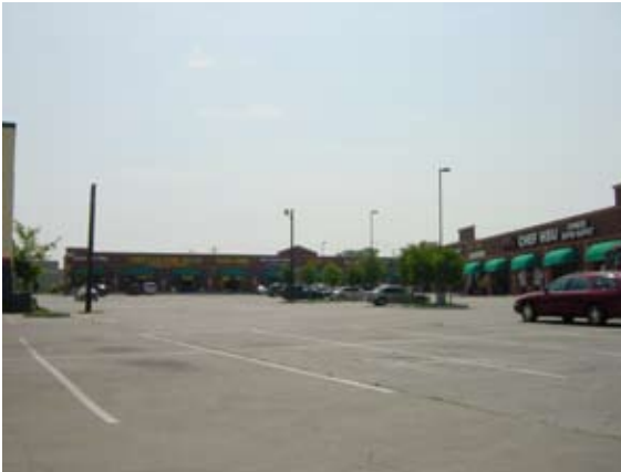
Streets lined with blank walls and parking lots feel unsafe and uninviting to pedestrians.
