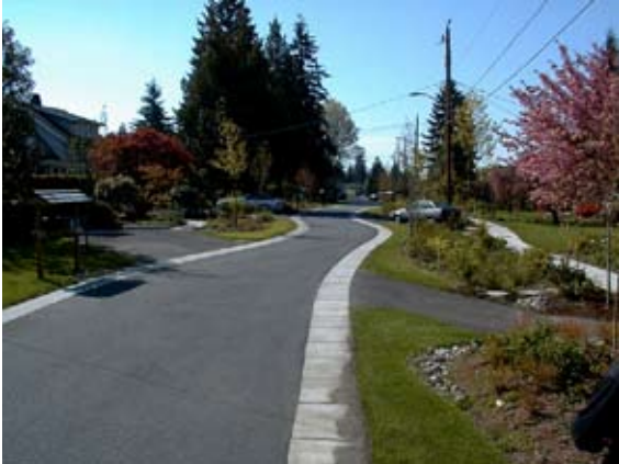
This example of a green street in a residential neighborhood employs natural vegetation to reduce the need for irrigation and absorbs area run-off without the use of storm drains.
