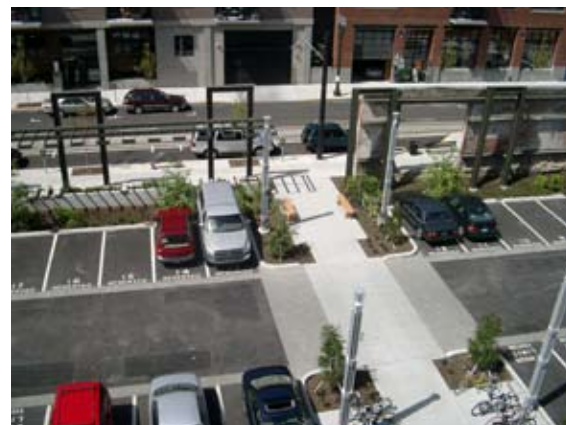
The use of permeable pavement in parking lots allows water to filter on-site. Additional run-off is caught by vegetated swales that separate the sidewalk from the parking area while also adding pleasant landscaping.
