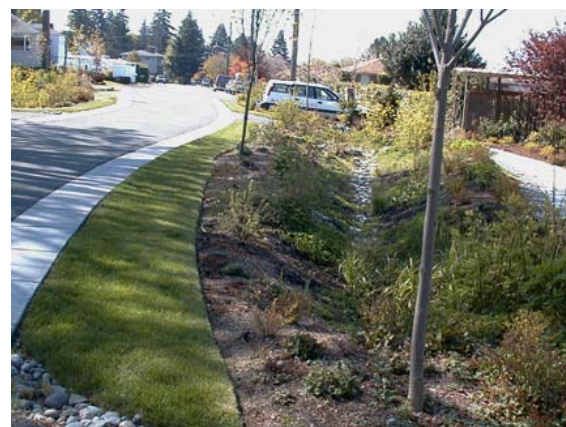
Storm water management techniques take many forms from vegetated curb cuts that absorb parking run-off to depressed vegetated swales that draw street and sidewalk run-off from neighborhood streets (above and below).
