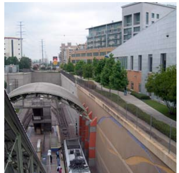
Reducing vehicle miles traveled includes bringing people closer to where they work and shop. ForwardDallas! will significantly direct new investment into transit oriented development areas such as Mockingbird Station where people can live, work and shop within walking distance of high-quality transit service.
