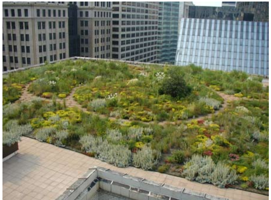
Rooftops present great opportunities for implementing green features such as an eco-roof. Chicago City Hall utilizes a green roof treatment in order to help curb the urban heat island effect.
