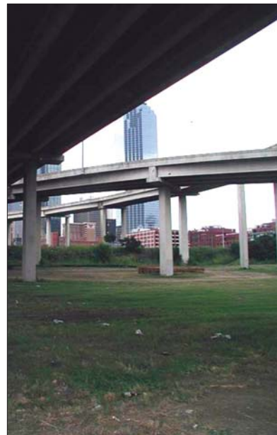
Existing Freeway Infrastructure
