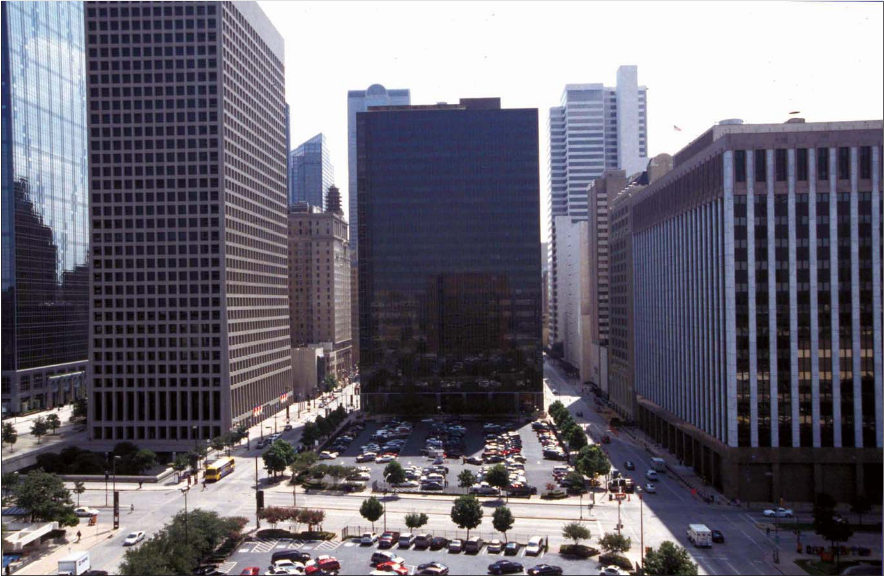
Aerial View of Griffin Street Garden Site from Across Griffin Street
