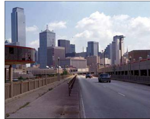
Existing Viaduct Cuts Across Site
