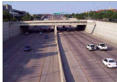
Existing depressed Woodall Rogers freeway
