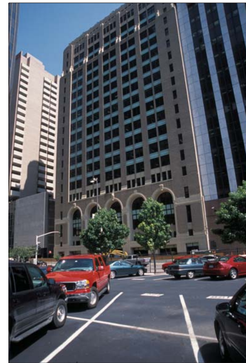
View Towards the Buildings to the South
