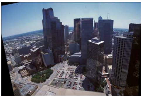
Pacific Plaza Existing Conditions
