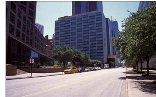
Existing Historic Structures on Site
