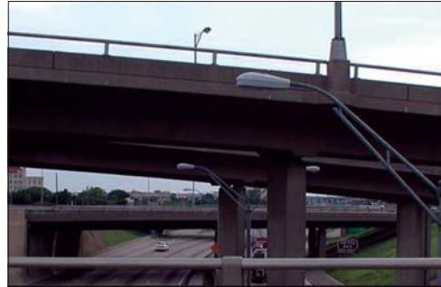
Existing I-30 Freeway Cuts Across Site
