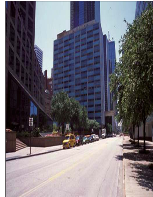
Existing Surface Parking Lot on Site
