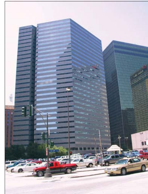
View Towards One Dallas Center
