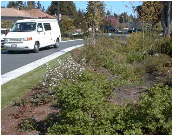
Innovative storm water management techniques use vegetated sloped swales that draw run-off from roads and filter pollutants on-site and through the soil.
