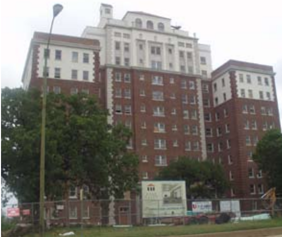
Oak Cliff condominium redevelopment.
