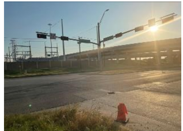
IH 35E Exit Ramp and Riverfront Blvd. — No Sidewalk on Southside of Riverfront Blvd.
