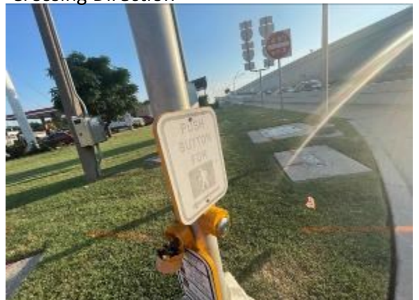
Riverfront Blvd. and Cadiz St., Southeast Corner Pedestrian Crossing Push Button Broken and Signs Need to be Replace and Repositioned for Proper Crossing Direction
