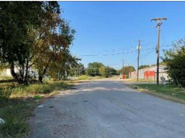
Driveway 2 at Dearborn St. and Rock Island St. Looking North
