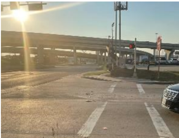
IH 35E Exit Ramp at Riverfront Blvd. — No Sidewalk West of Intersection
