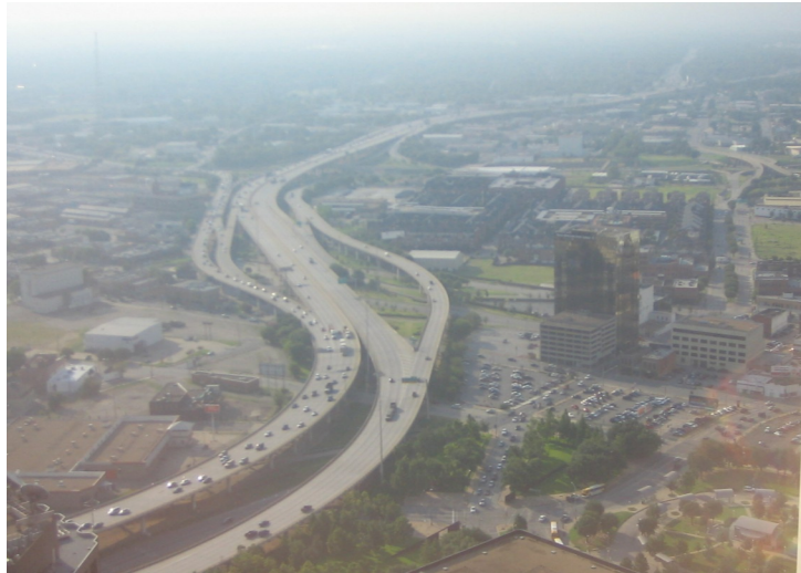
Figure 9 - Stemmons Freeway as seen from Downtown
