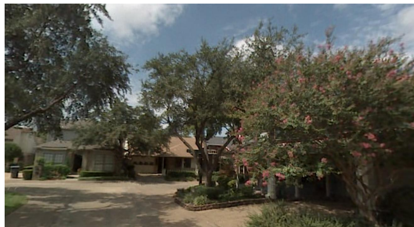
Figure 28 - Small-lot residential development is a development pattern which can increase density as redevelopment occurs in the neighborhood near the DART Green-Line Market Center Station. This development should encourage connectivity and walkability, offering short blocks and tree-shaded walkways connecting to area amenities.
