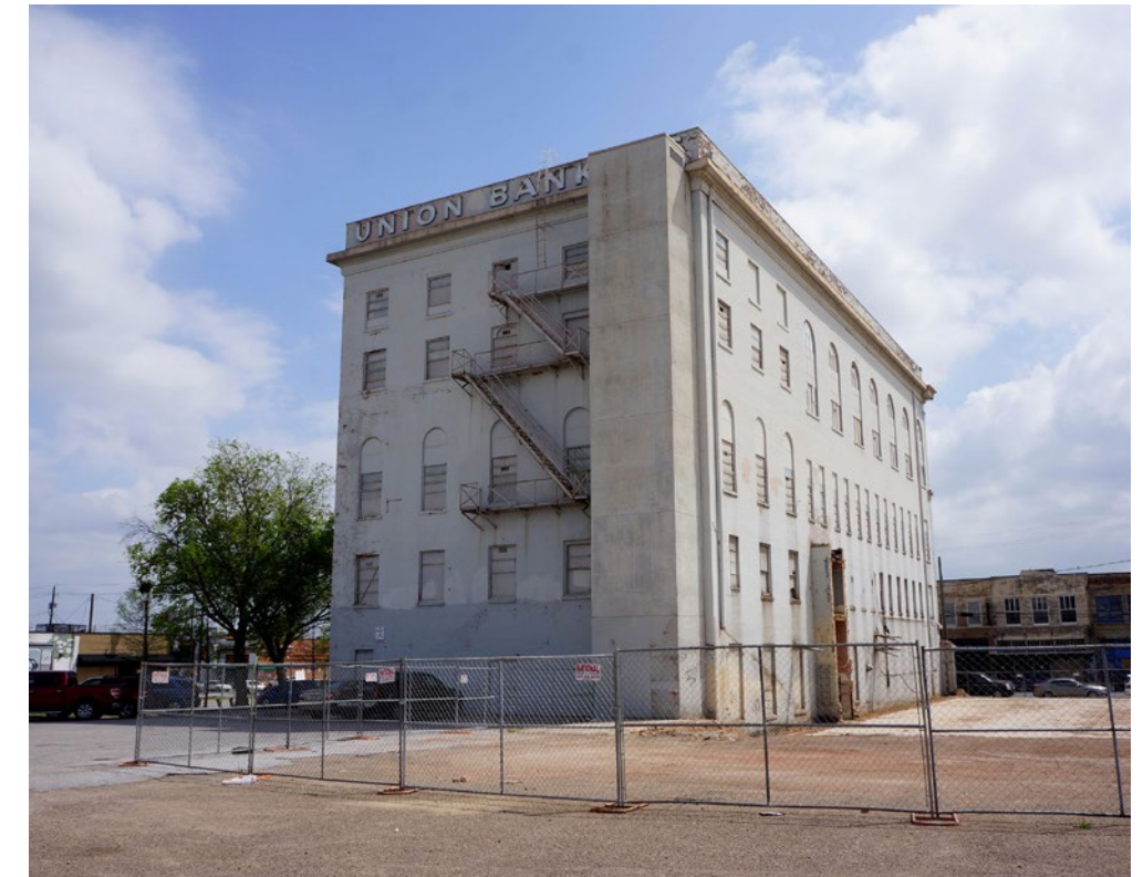
View of north facade
