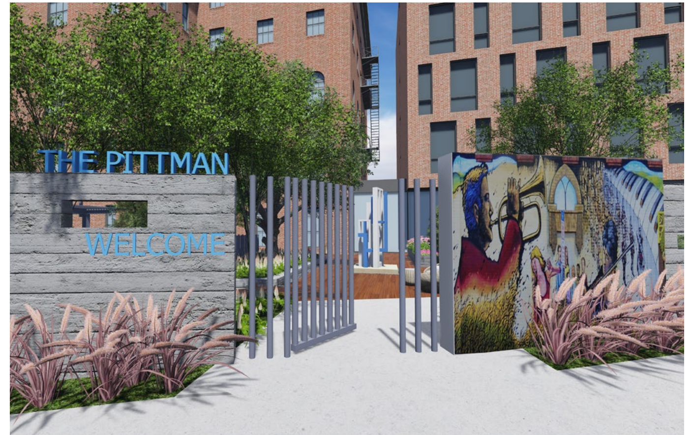
View of art wall and patio entry gate along Elm St.
