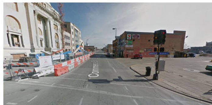
STREETSCAPE FROM HARWOOD & COMMERCE LOOKING EAST
