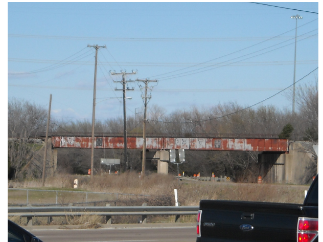
Figure 4.11 (Top) Existing Area 4 Development
