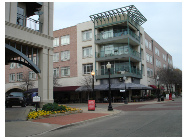
Figure 4.2 (Top) Existing Area 1 Development - Garland Road at Gaston Avenue
