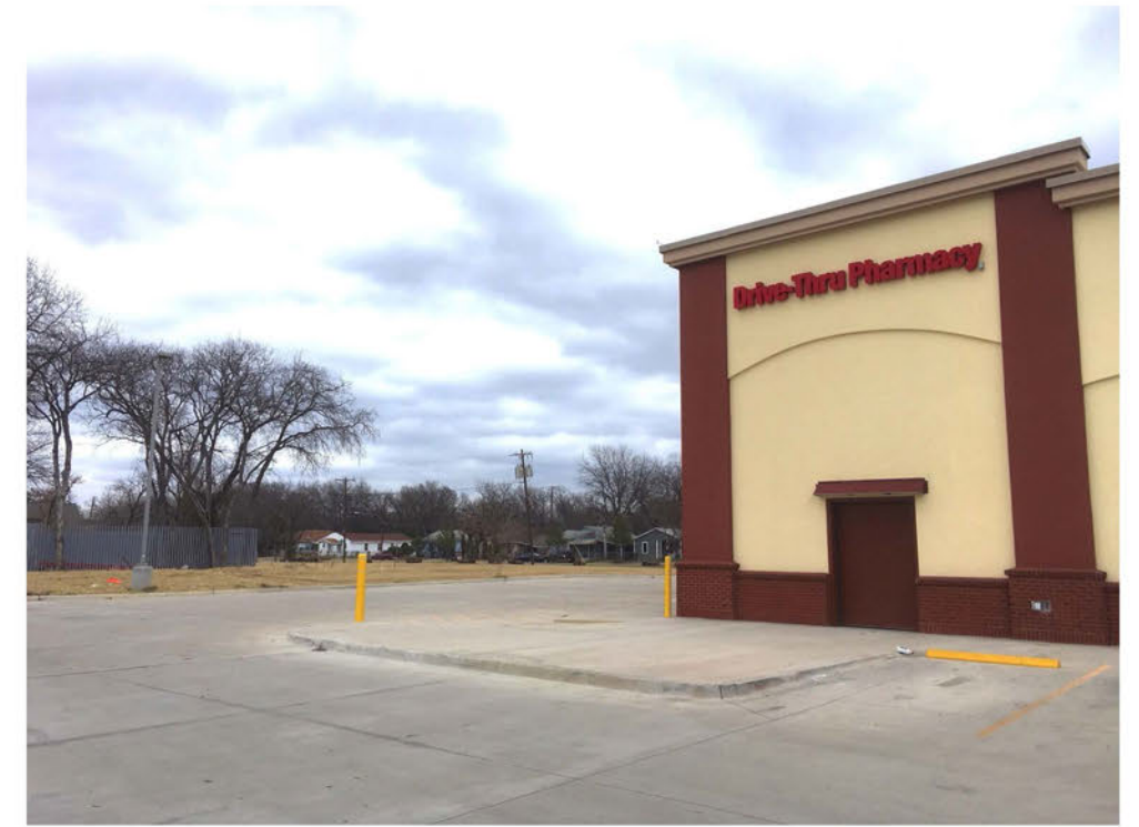
8 View of site from Sylvan
