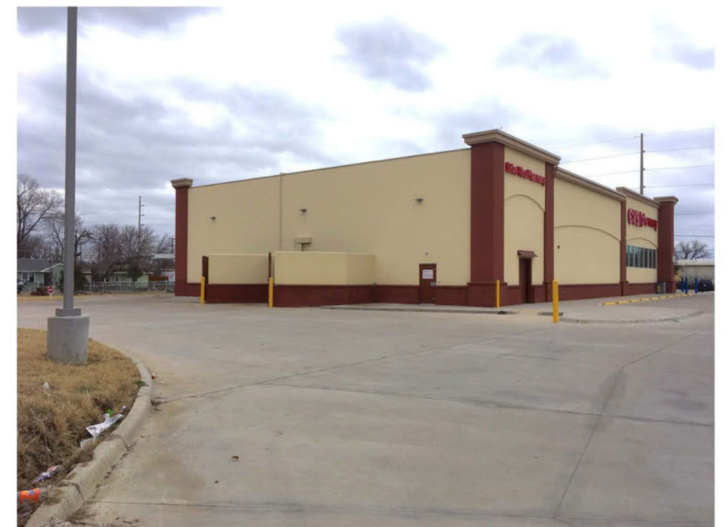
9 View from site looking South
