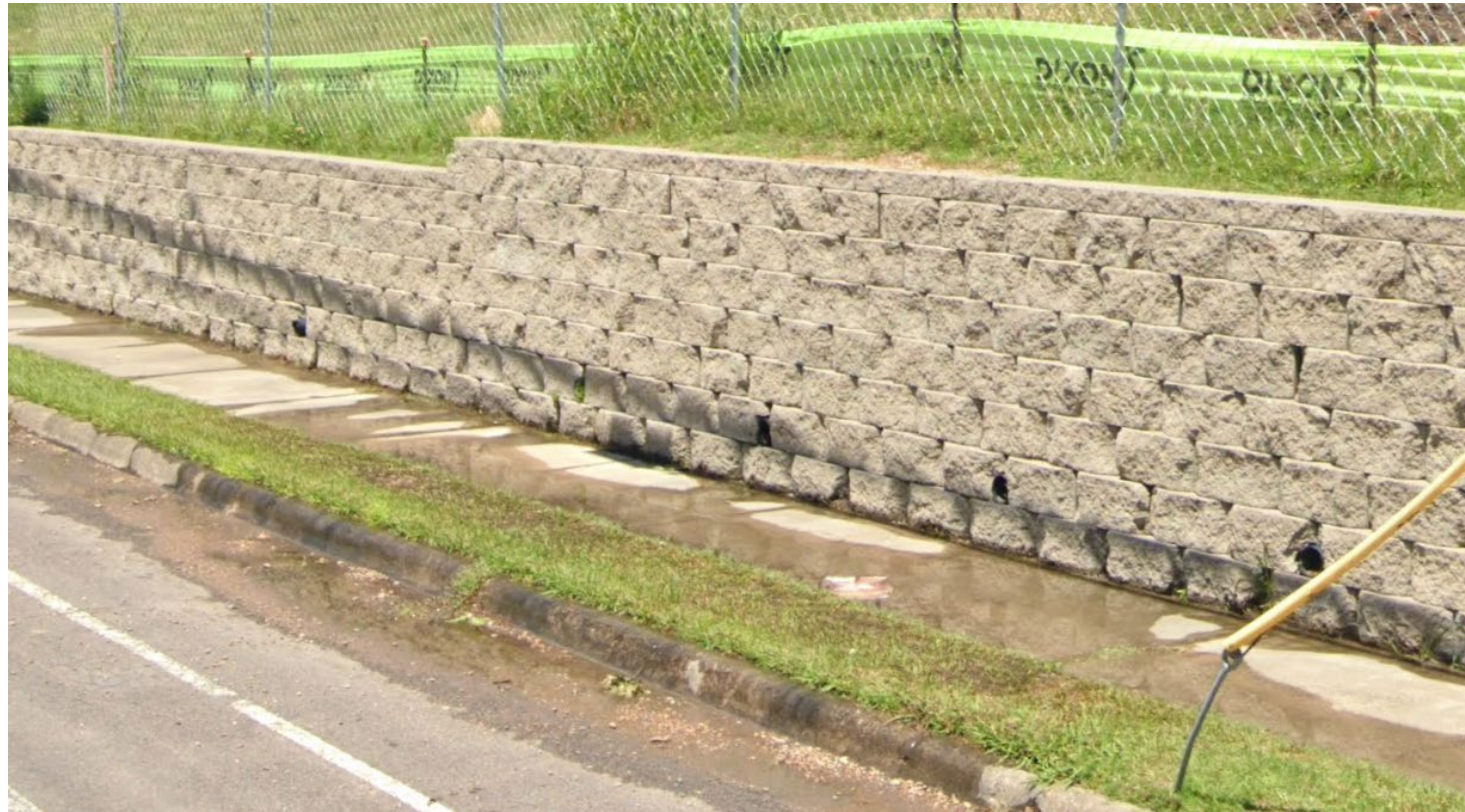
Rosemont Upper School 179 N Montclair Avenue (View from Mary Cliff Rd.)
