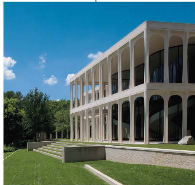
Beck Residence Dallas TX 1964
