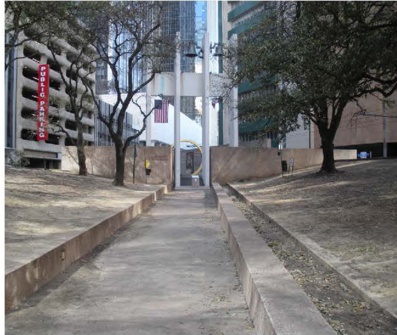
Exposed Soil Due to Overuse and Shade
