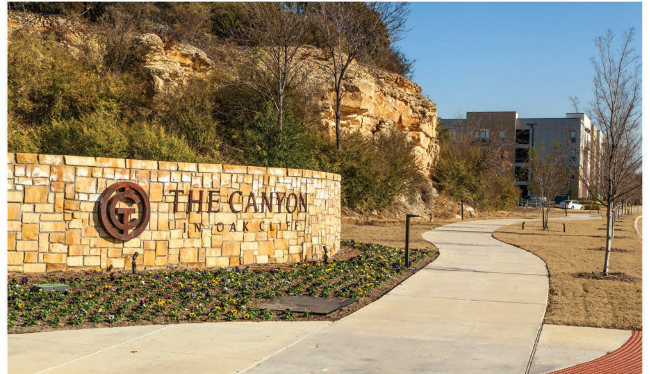
VIEW OF GATEWAY WALL AT HILLSIDE DEVELOPMENT
