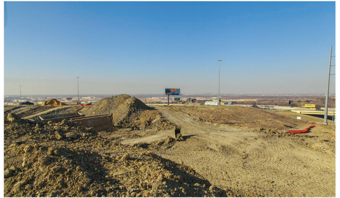
VIEW LOOKING NORTH FROM WESTMORELAND
