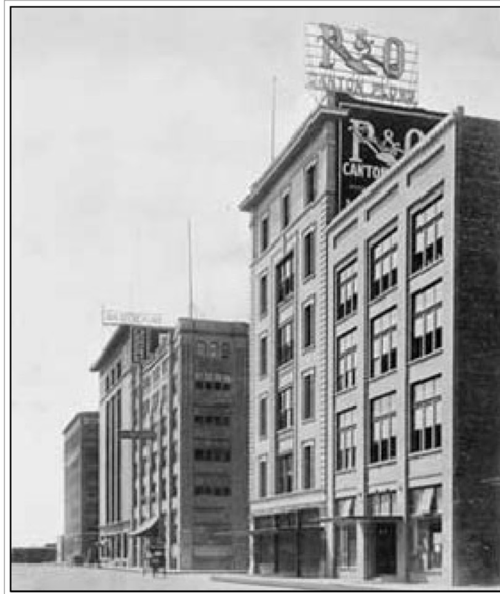
LOOKING NORTH WEST
