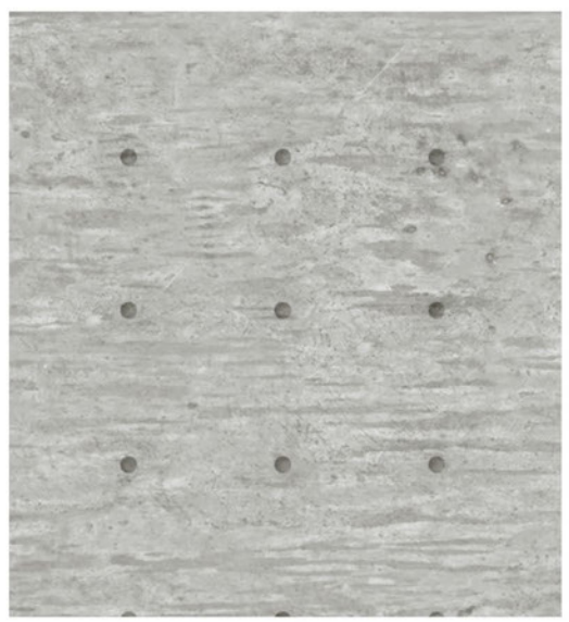
Site Retaining Walls (Exposed Concrete)
