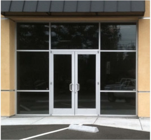
Storefront System (Anodized Aluminum)
