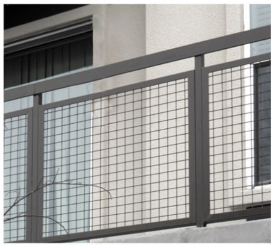
Balcony Handrails (Painted Steel—Warm Gray)
