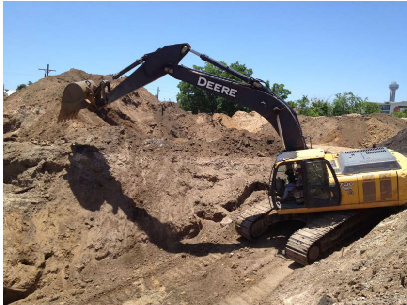
WASTEWATER SIPHON EXCAVATION
