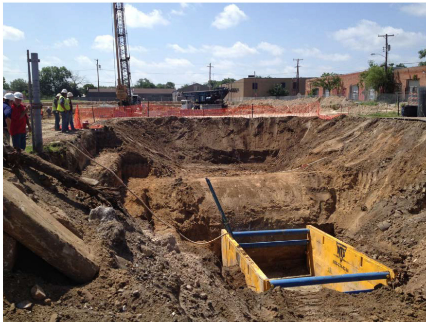
EXCAVATION UNDER 18' HORSESHOE STORM
