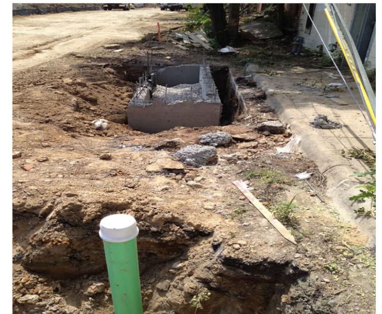
NEW STORM INLET AND WASTEWATER LATERAL
