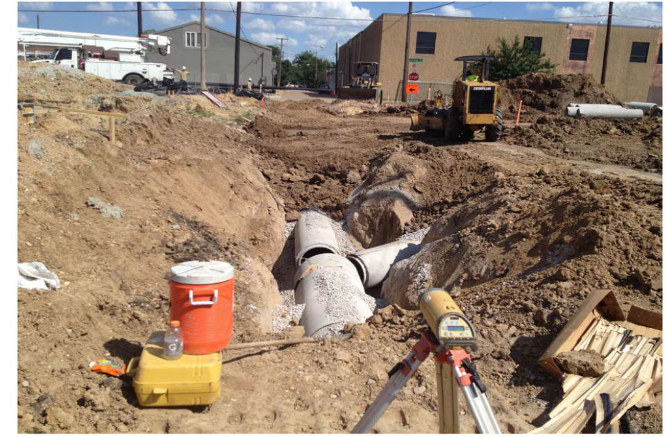
NEW STORM LINES ON GOULD STREET
