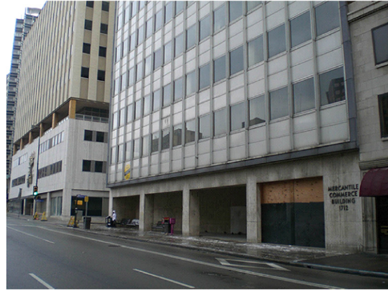
VIEW SOUTHEAST ACROSS COMMERCE STREET
