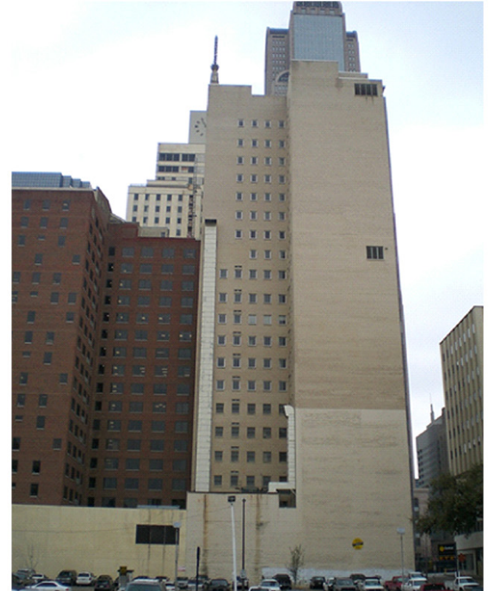
VIEW NORTH OF SOUTH ELEVATION
