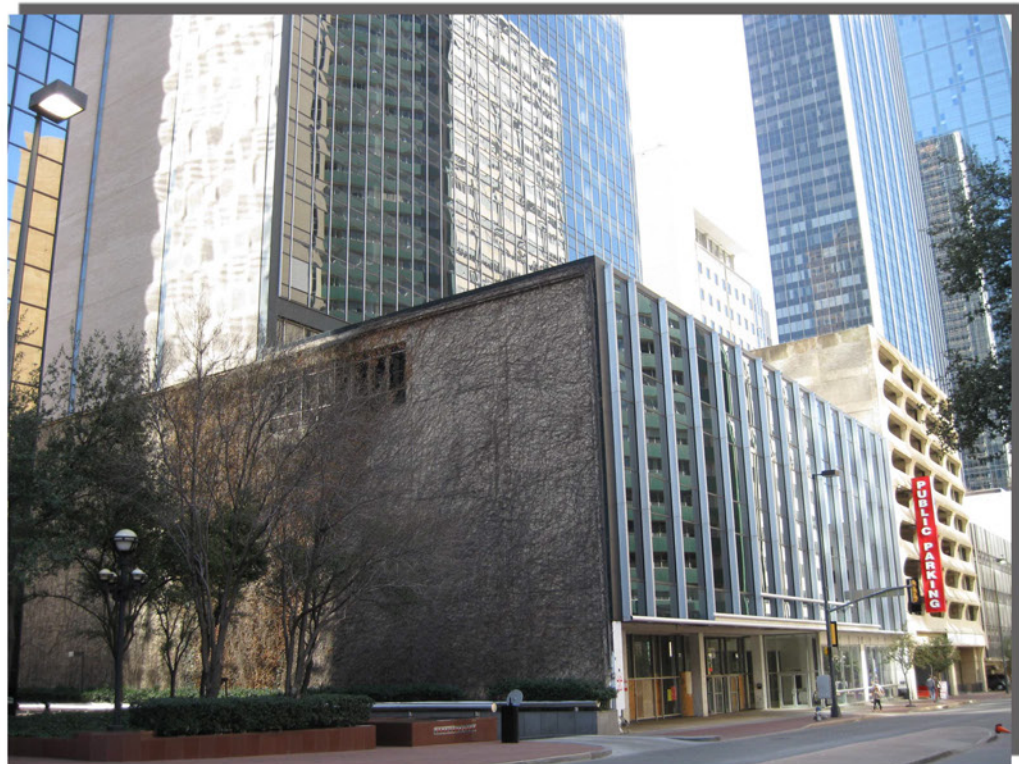
VIEW OF THE PACIFIC STREET FACADE LOOKING WEST
