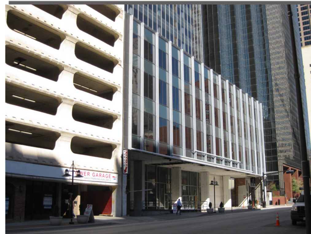
VIEW OF THE ELM STREET FACADE LOOKING EAST
