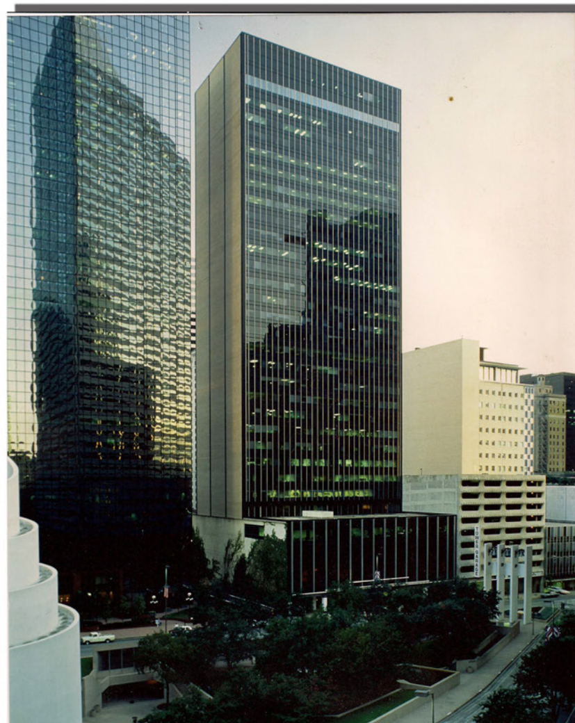
VIEW OF THE NORTH FACADE LOOKING ACROSS THANKSGIVING SQUARE
