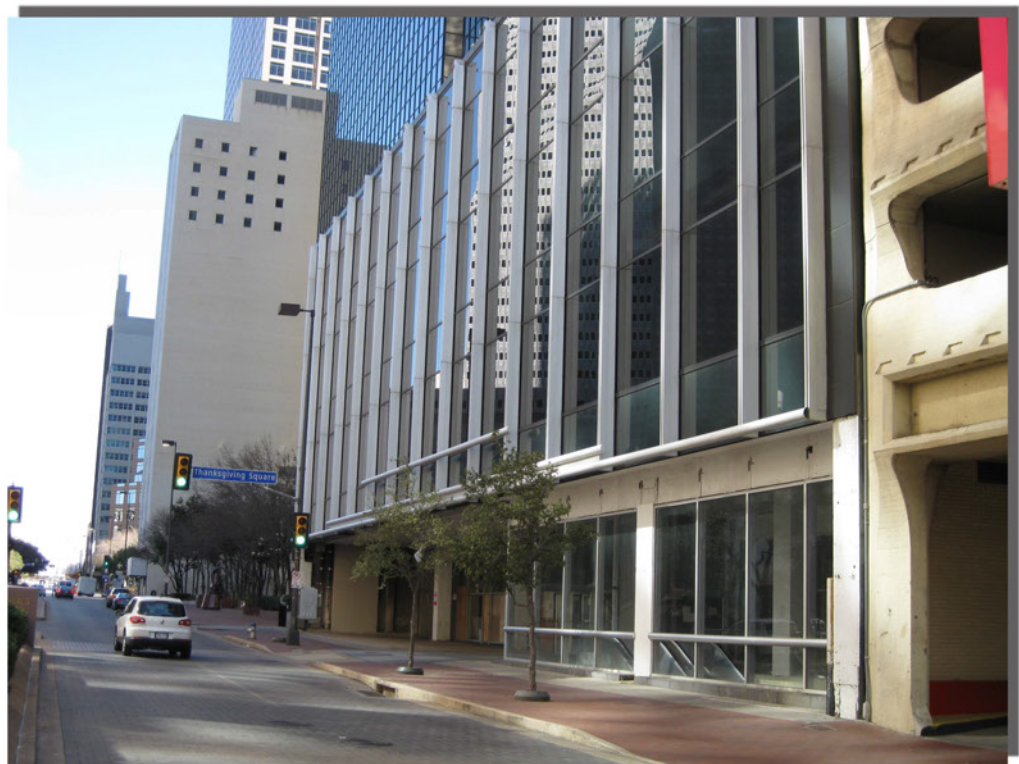
VIEW OF THE PACIFIC STREET FACADE LOOKING EAST
