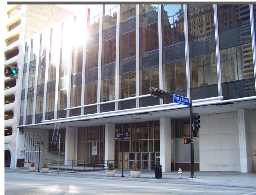
VIEW OF THE ELM STREET FACADE LOOKING WEST
